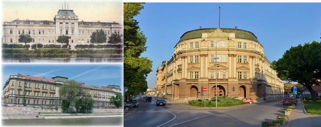
Fig. 3. Three major phases in the construction of the building: The original building, consisting of two tracts with ground floor and first floor, from 1886 (up left); After the First World War, in 1925, the building has been extended for one more floor (down left); Main entrance to the part of the building used by the University of Niš (right)
