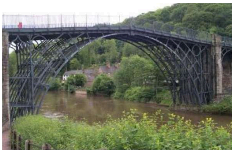
Фигура 1. The Iron Bridge in Coalbrookdale, UK [5]
