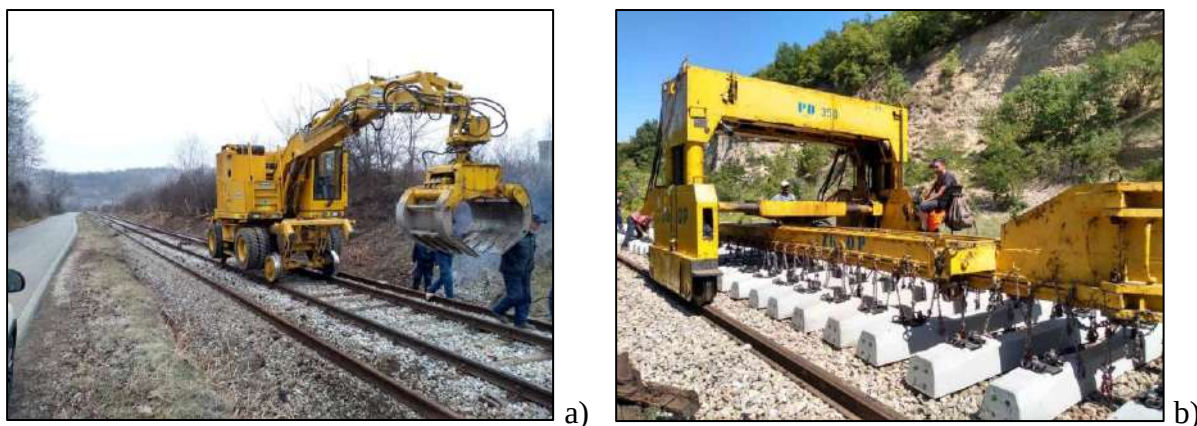
Figure 2. a) old track removing; b) laying new sleepers using a gantry crane PD 350 (photos by M. Milijić)
