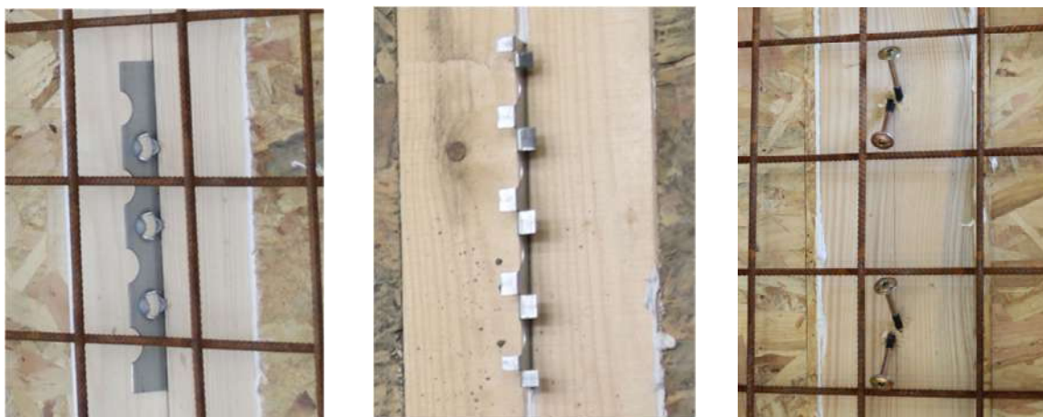
Figure 2. Connectors installed in the timber part of the cross-section before concreting: pressed punched metal plates (left), glued metal plates (middle) and screws with plate-shaped heads (right)
