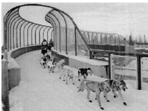
Figure 19. Tudor Road, pedestrian Bridge [17].
