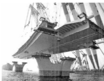
Figure 4. Trans-Tokyo curved orthotropic exit ramps – high level bridge installation was with floating cranes. Photo by Owners
